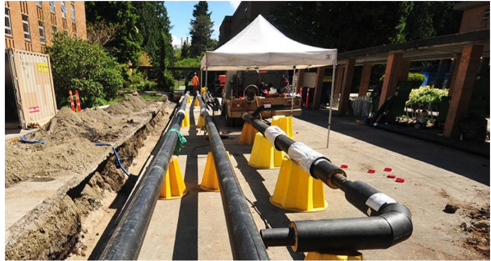
Pipes going in at University of British Columbia. Photo by UBC
