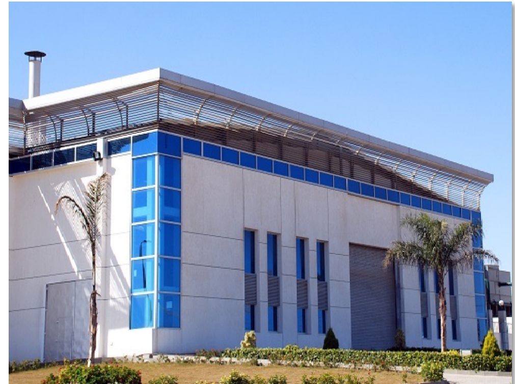
Smart Village, Egypt's first DC project
